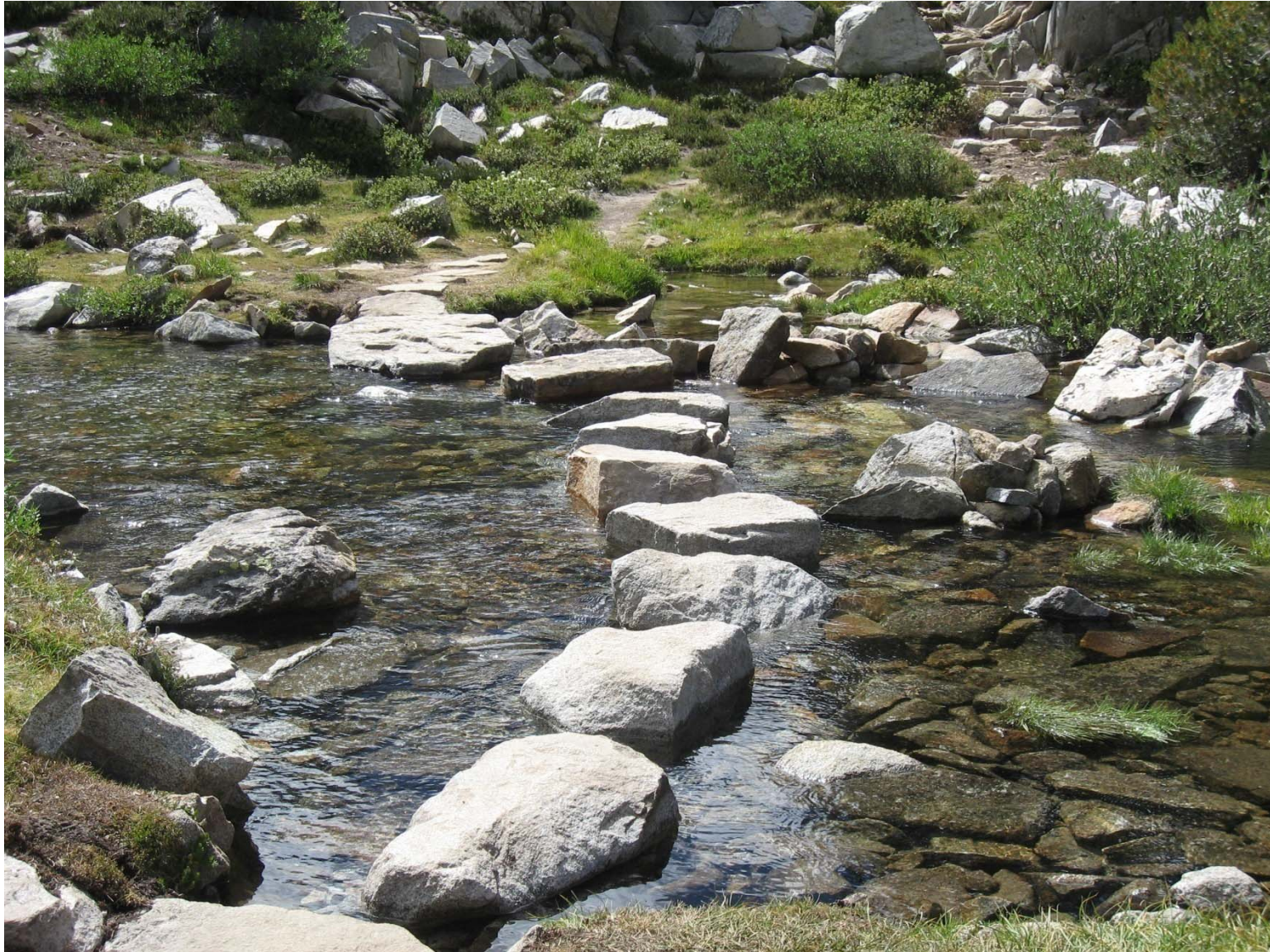
A well-designed stream crossing, with flat-topped stepping stones
